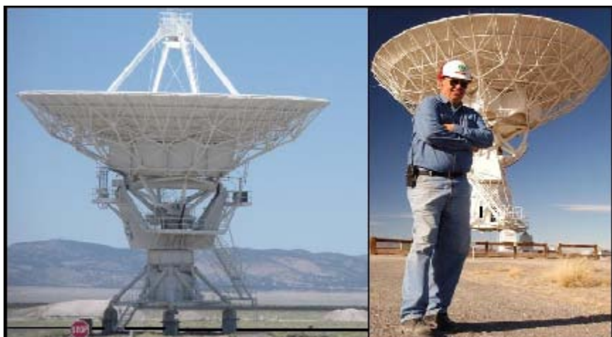
Jon Spargo, Safety Officer, Astronomer, And Lifelong Rail Fan: Yep, the line at the bottom of the antenna in the left image is a rail line—actually double tracks that are used to move the giant antennas. Jon still combines both childhood hobbies.
